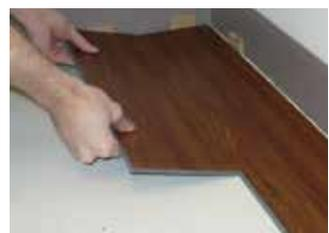
Install the long side of the first plank of the second row. Remember to place a 1/4 inch (6.3mm) spacer between the wall and the short side of the plank. Insert the tongue side into the groove side of the previous row at a low angle and rotate downward until plank is flat with the substrate.
