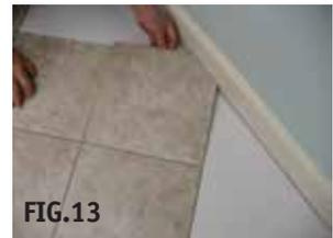
Fitting tile around door mouldings, pipes or irregular shaped walls can be done by direct scribing. Whenever possible, undercut door mouldings the thickness of the tile to allow tile fit underneath door mouldings. Heat the back of the tile and cut along the scribe or pencil mark on the pattern side of tile.
