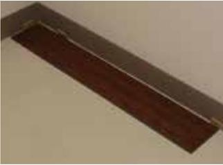
Begin laying planks from the left side of the starting wall and work to the right side. The tongue side of the plank shall face the starting wall.
