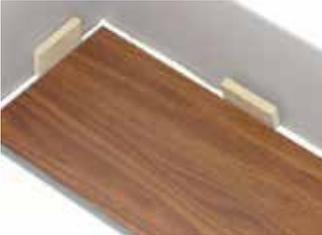
Place 1/4 inch (6.3mm) spacers between the short and long side of the planks and the wall. Always position one spacer between the wall and where the planks join.
