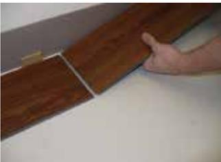
The end joints of the planks in the first row are assembled by inserting the tongue side into the groove side of the previous plank at a low angle. Gradually lower the plank down flat until the end joint closes, insuring that the planks are perfectly aligned. Install remaining full planks in the first row.
