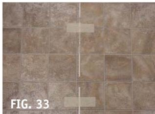
**FIG. 33:** After the exact pattern match has been achieved, place masking tape at seam overlap to prevent flooring from moving. Fit second piece of flooring around the perimeter of the room.
