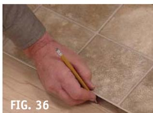
**FIG. 36:** Mark substrate along seam edge with a pencil. Do not contaminate seam edge with lead from pencil.
