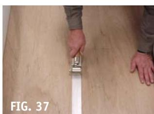
**FIG. 37:** Fold back each sheet of flooring at the seam area to expose each adhesive line. Apply Tarkett S-860 Seam Tape to the substrate, so that it is centered over the pencil line. Roll seam tape in place with a hand roller.
