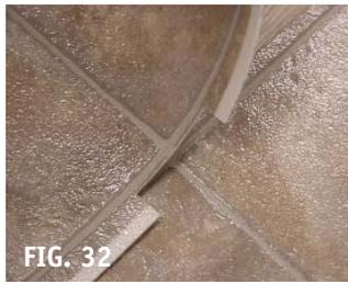
**FIG. 32:** In order to obtain the proper overlap of the selvage edges, make a cut out or window on the outside edge of the grout line along the factory edge. Make one cut out every few feet depending on how long the seam is. These cut outs will allow you to properly align the grout lines at the seam overlap.
