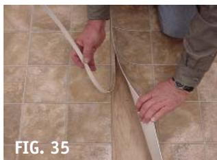
**FIG. 35:** Lift top edge of flooring and carefully remove bottom salvage piece.
